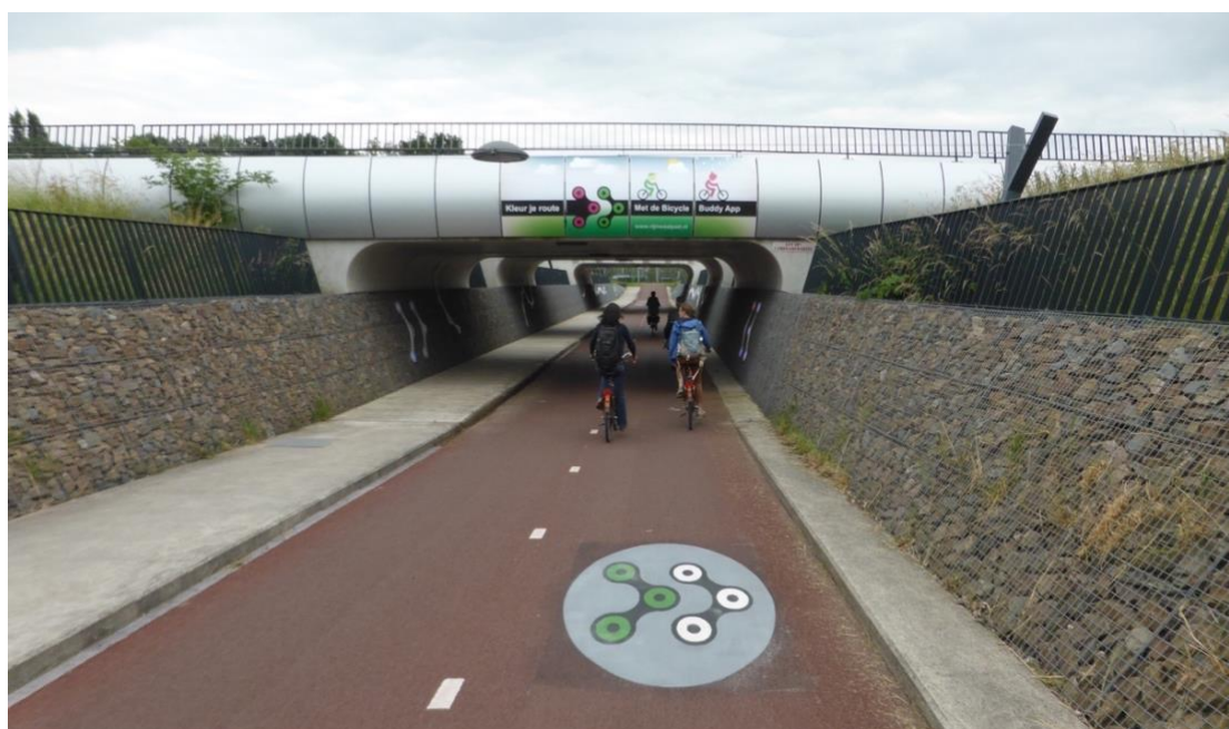
Figure 44 A semi-submerged tunnel under an A-road on a national cycle route in the Netherlands. The retaining walls are designed open outwards to allow for lots of natural light and clear sight lines to the far side © Interreg North-West Europe CHIPS
